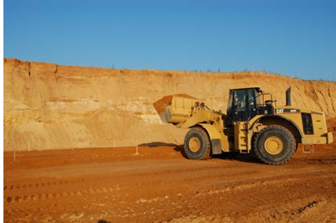
Figure 3.3 Placing the fill material with a Caterpillar 980H bucket loader (Tehrani 2009).
