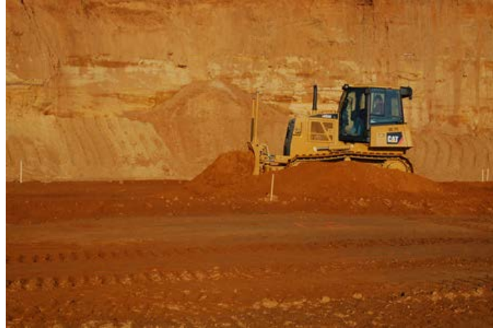
Figure 3.4 Spreading the fill material with a Caterpillar D6K bulldozer (Tehrani 2009).
