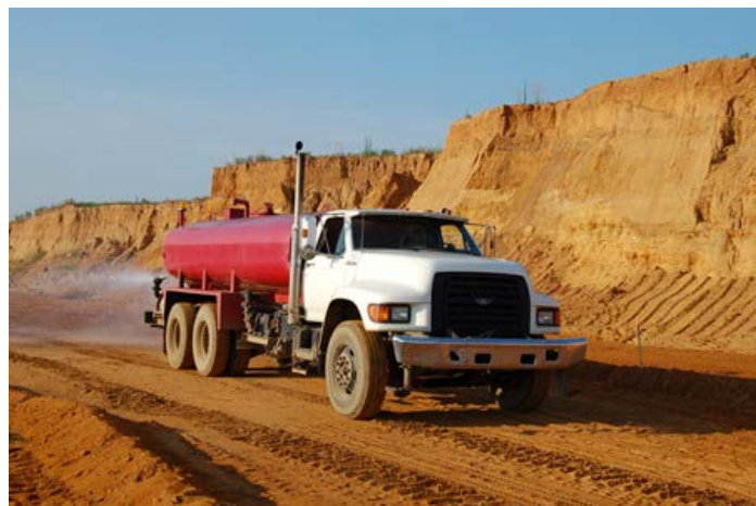
Figure 3.5 Moisture content conditioning of fill material before compaction (Tehrani 2009).
