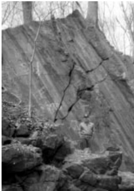
Figure 24. Wooddale railroad cut, steep fault surface on the west wall of the cut.
