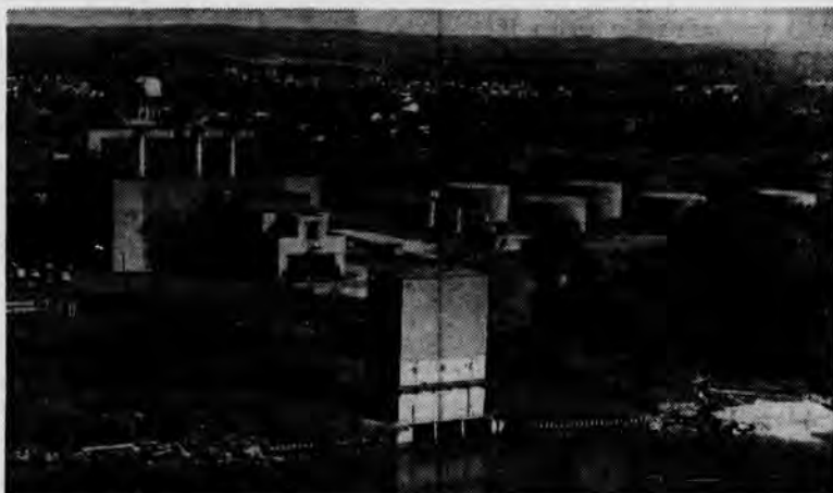
Andrew Willgoos Turbine Laboratory where jet engines and their components are explored. Cooling water from the Connecticut River can be pumped through a maze of conduits at the rate of 160,000 gallons per minute — 3½ times the consumption of a city of half a million people.
