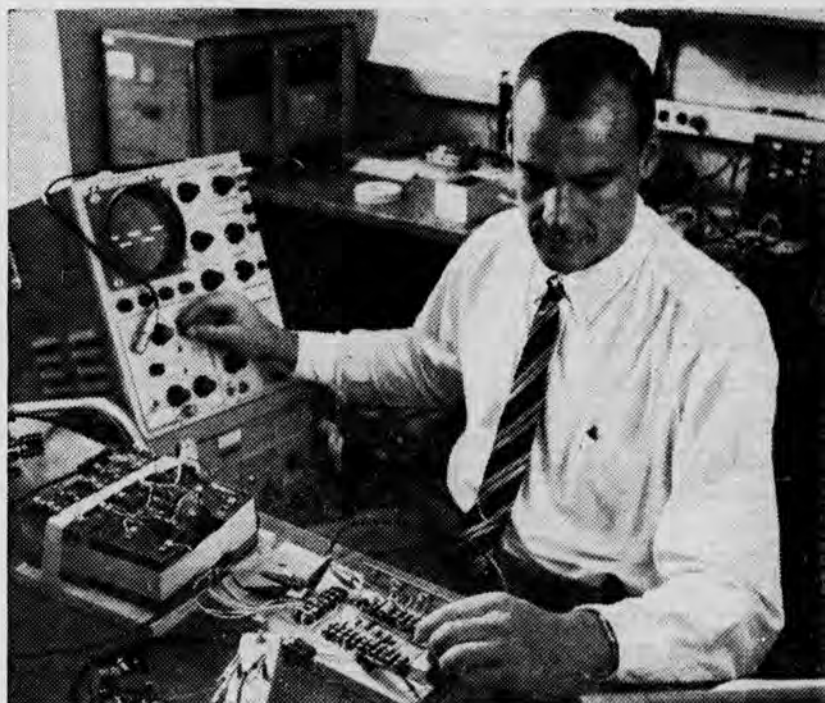
Dick Abraham of Bell Telephone Laboratories, here experimenting with closing the loop on a transistor feedback amplifier.
