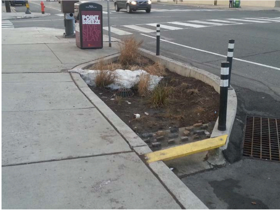
Figure 2.9 Existing curb extension on West Washington Avenue, with stormwater planter.
