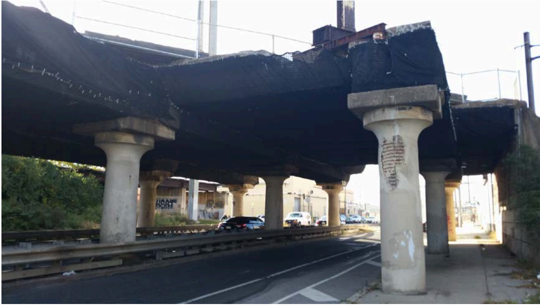
Figure 1.4 The elevated rail that crosses Washington Avenue at an angle at 25 th Street, built in 1925. The black netting is for catching falling concrete debris, because the structure is in need of repairs.
