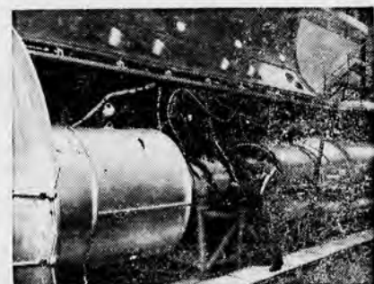
In chambers like this at the Willgoos Turbine Engine Test Facility full-scale engines may be tested in environments which simulate conditions from sea level to 100,000 feet. Mach 3 conditions can also be simulated here.
