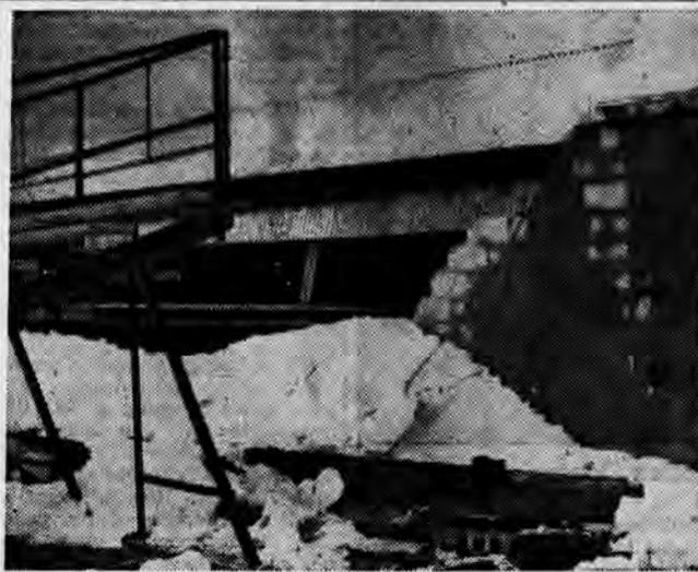
**WALL CRUMBLES** — Pictured is a view of the hanger at the east end of Carpenter Field House after the recent snowfall. The wall toppled because of heavy pressure on it from the snow. Spring practices, held in the hanger, were delayed while adjustments were made.
