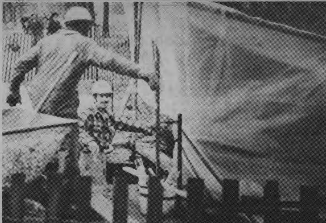
MAINTENANCE MEN FILL in the holes in front of Sharp Hall which had been dug to connect utility lines.
