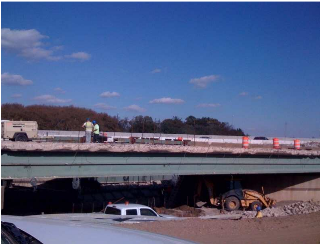
Figure 2.5 Photo of middle span w/ parapets removed
