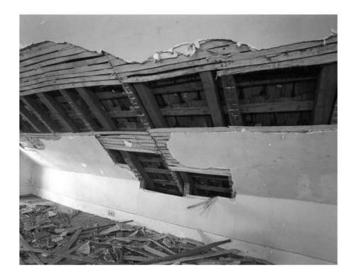
Figure 60: Reynolds House, second floor, Period I/II section: detail of roof framing in north wall.
