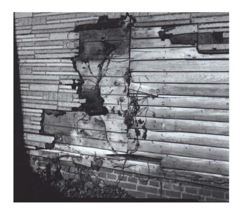
Figure 52: Reynolds House, detail of south elevation of Period III block, showing filled opening for earlier door.
