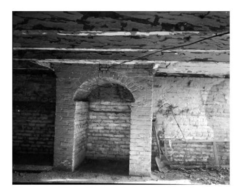
Figure 53: Reynolds House, cellar, relieving arch on east wall looking east.
