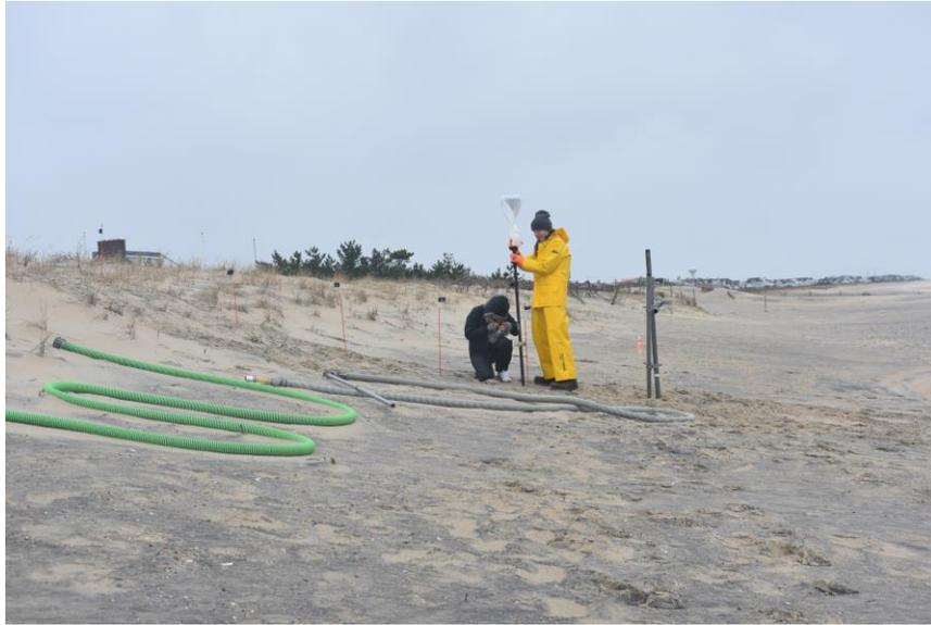
Figure 15 Surveying additional Data points with Leica GPS
