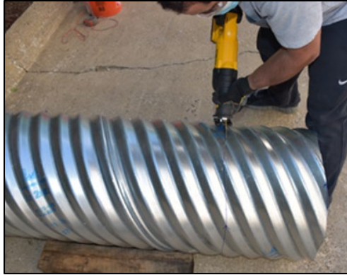
(a) Cutting the host pipe.
