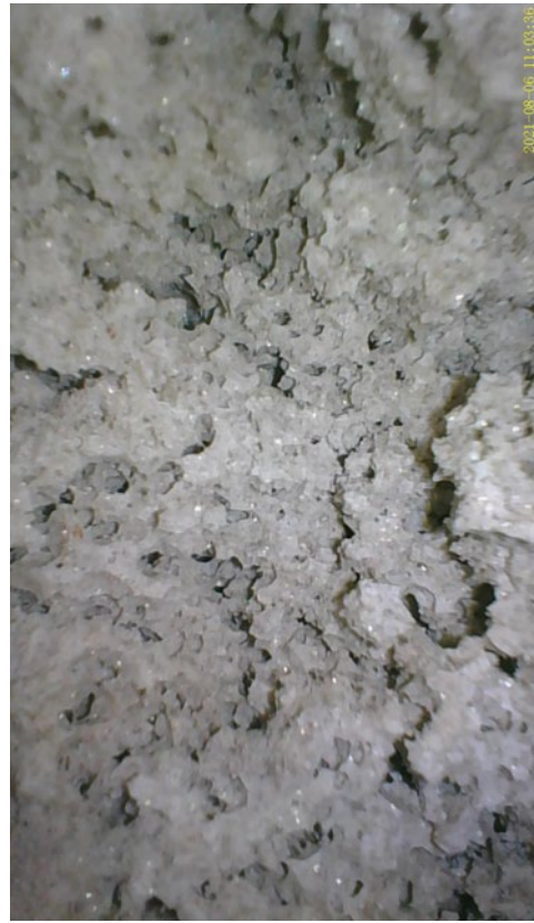
(c) Delamination (left: at the liner pipe; right: at the host pipe)
