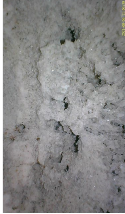
(c) Delamination (left: at the liner pipe; right: at the host pipe)
