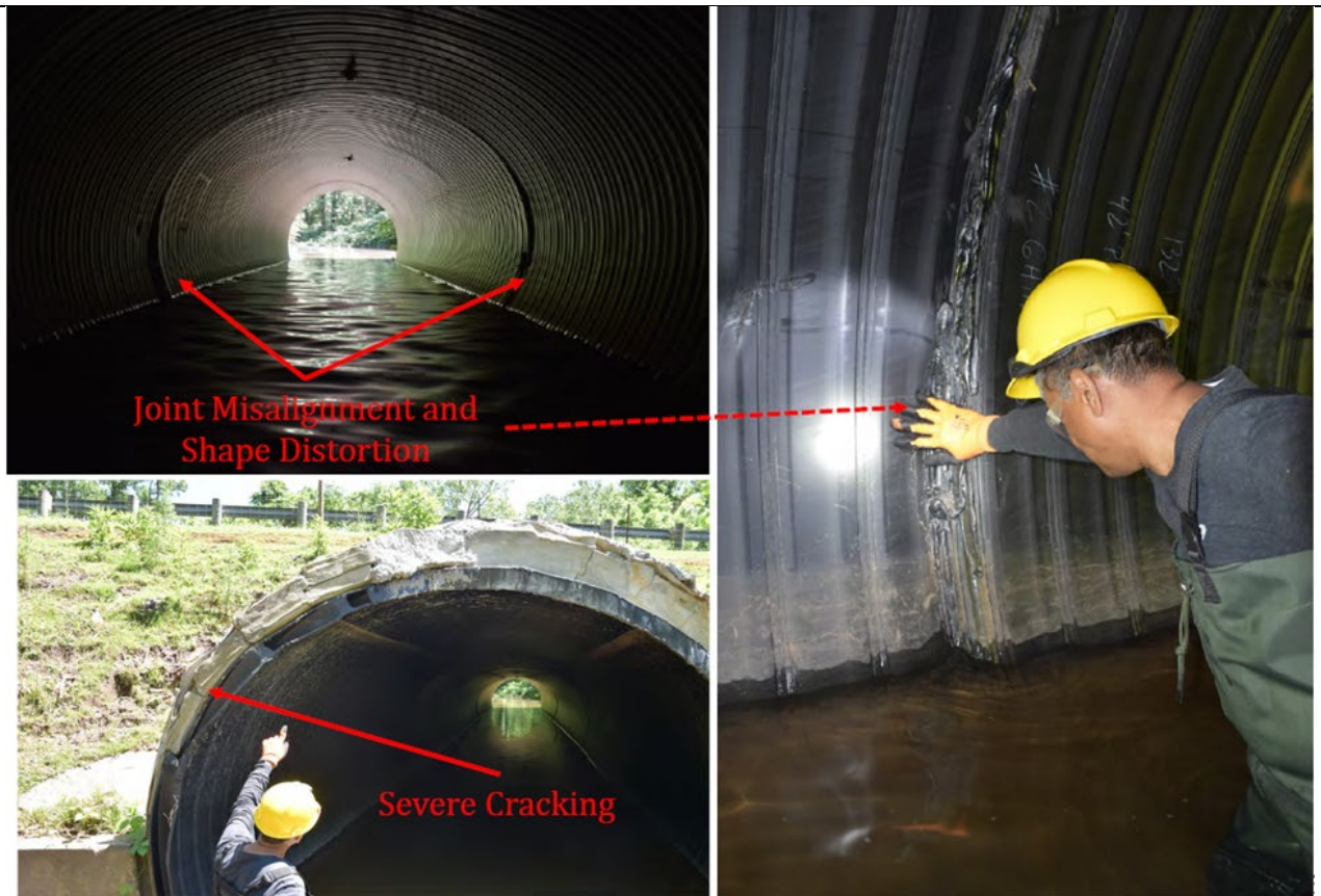
Several Cracks at the Bulkhead and Shape Distortion
