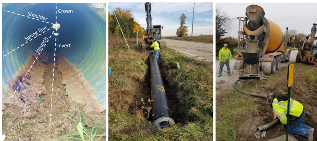
(a) Corroded corrugated steel pipe
