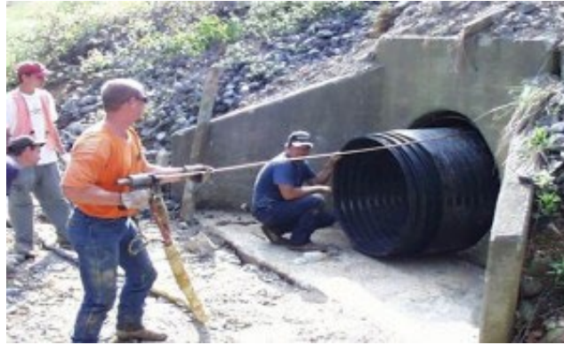
Figure A.12: URETEK team works to inject grout in between the pipes (Armstead 2015).
