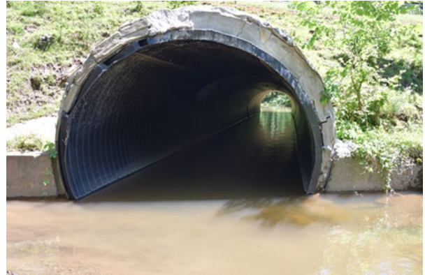
(b) Polyethylene Double-Layered Pipe
