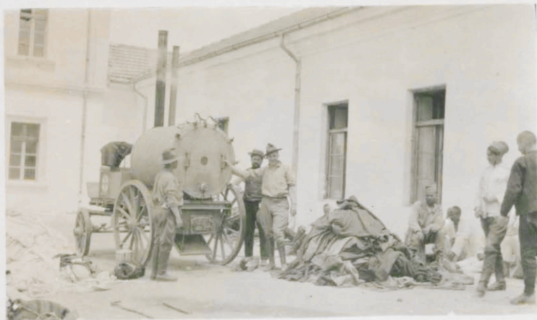
Steam Sterilizing bedding after sulphur fumigation at Prishtine Barracks.
