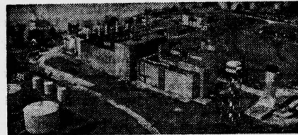
The Willgoos Turbine Engine Test Facility is the world's most extensive privately owned turbine development laboratory. Designed and built specifically to test full-scale experimental engines and components in environments simulating conditions at extreme altitudes and speeds, it is currently undergoing expansions that will greatly increase its capacity for development testing of the most advanced forms of air breathing systems.
