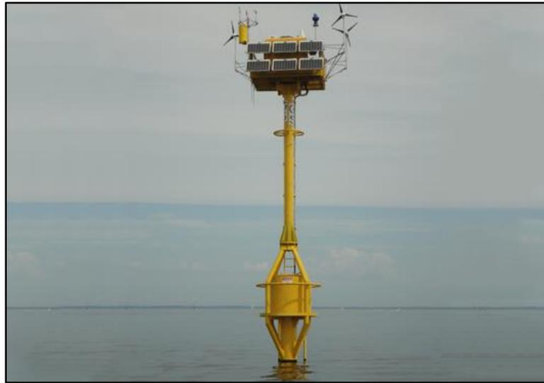
**Figure 18-New Jersey Offshore Research Device (NJORD), built by SEAROC, supporting a ZephIR 300. Reprint courtesy of SEAROC**
