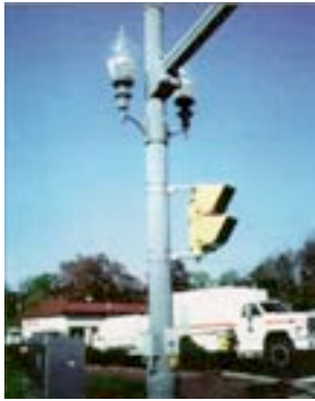
Figure 12 Integrated Pole with Acorn-Style Lighting
