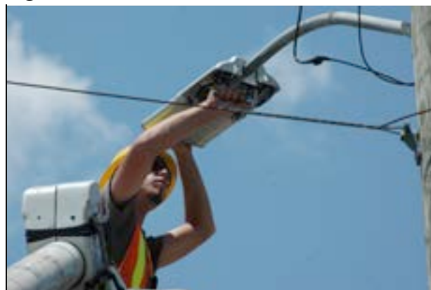
Figure 8 Asheville City Worker Installing LED Light Source: City of Asheville, NC
