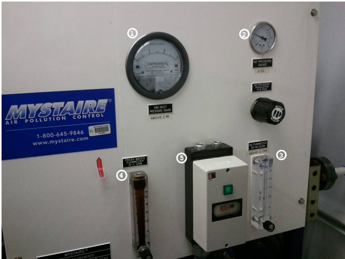
Figure 5.7 Front panel of the ICP scrubber: 1 differential pressure gauge, 2 nitrogen pressure gauge, 3 nitrogen flow meter, 4 freshwater flow meter, 5 power switch.
