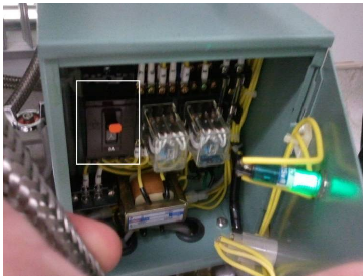
Figure 6.3 Inside of the filter control, showing the breaker with the orange mark on the switch.
