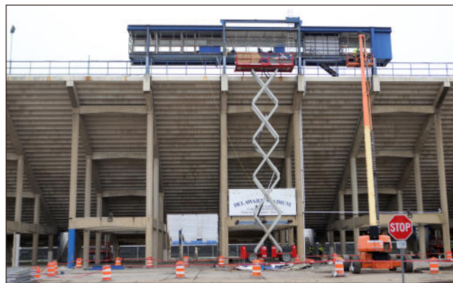
A demolition crew takes down the old press box at Delaware Stadium, which is undergoing renovations.
