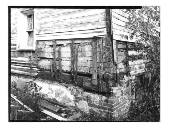
Figure 84: Simmons Farm House, detail of log construction on the south corner of the Period I section showing foundation with brick repair, looking north.
