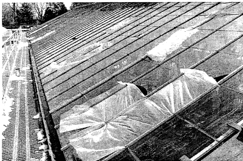
Figure 5.27 Plastic Sheets Temporarily Replace the Glass Panels that Cracked and Fell Out As a Result of the Fast Accumulation of Heavy Snow (Photograph courtesy Longwood Gardens, Inc.)
