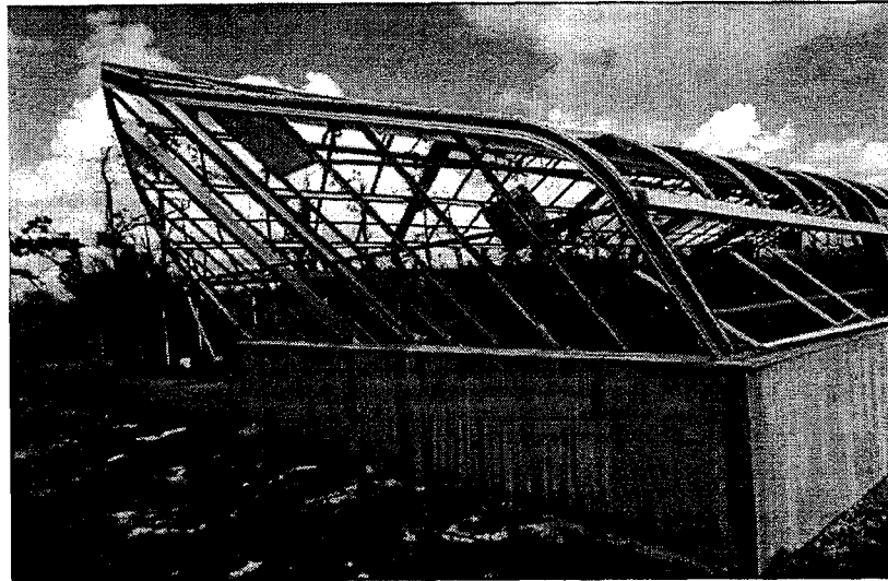
Figure 5.4 Tilting of Aluminum Frame Greenhouse in Hurricane Andrew's Aftermath. (Photograph courtesy Fairchild Tropical Garden.)
