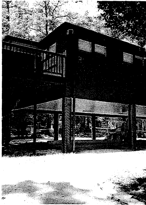
Figure 5.32 Past Flooding Experiences Led to Construction of an Administrative Office Set Upon Eight-Foot Pylons (Photograph by author)
