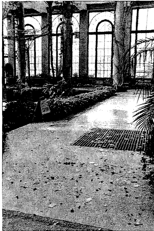
Figure 5.28 Shattered Roof Glass Plummeted to the Conservatory Walkways and Planting Beds (Photograph courtesy Longwood Gardens, Inc.)
