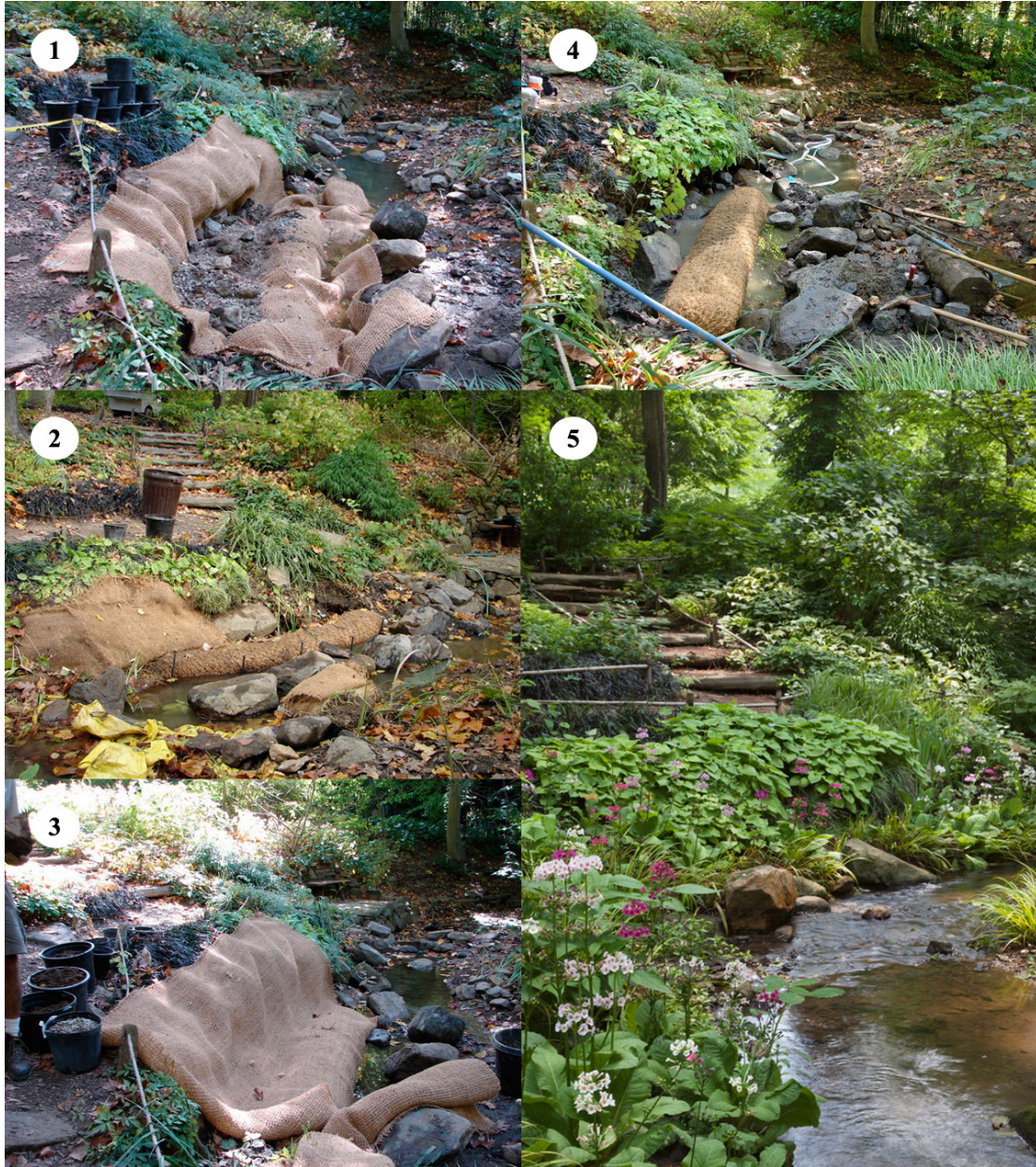
Figure 26 Stages of coir log installation for erosion control and stabilization of the Bells Run Creek at Chanticleer: 1. Filling fabric, 2. Fabric over coir log and on bank, 3. Fabric and coir log pinned in place, 4. Coir log, 5. One year later (provided by Chanticleer).
