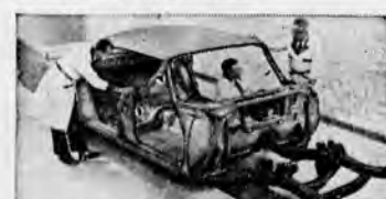
UNIBODY Construction: frame flows into the body, makes it twice as strong, twice as quiet—surrounds you with silent strength.
